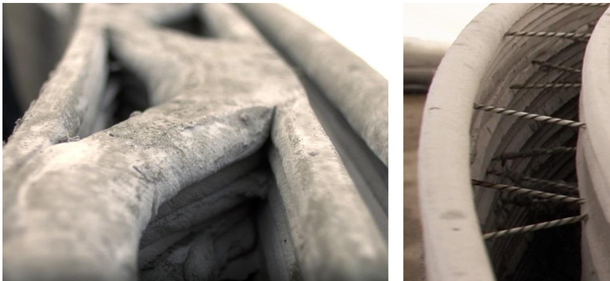
Fig. 1. “Printing” of a wall by additive techniques
