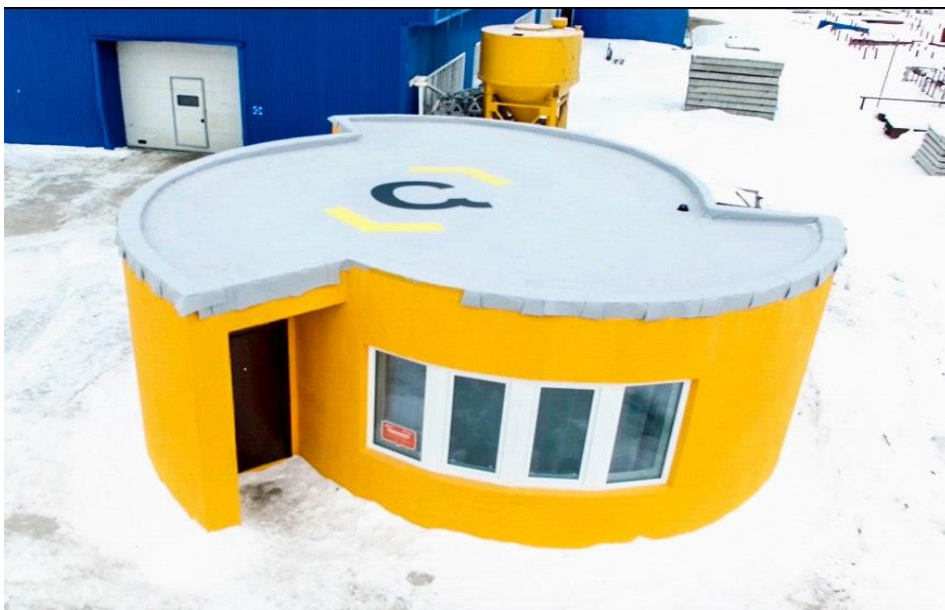
Fig. 4. A house printed by the additive technique in Russia
